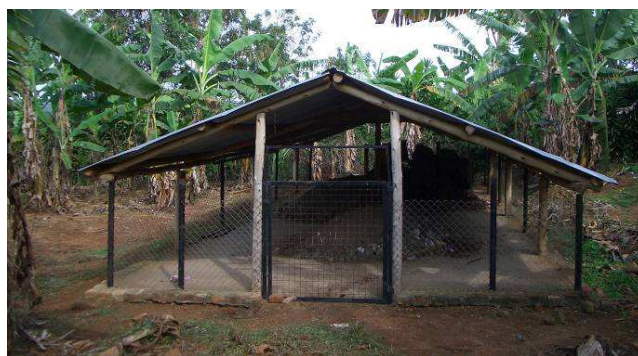
Figure 3: Drying shed for faecal matter from UDDTs at Kalungu School, Uganda. The caretaker has to take the containers with faeces from the UDDTs to this shed (source: EcoSan Club, 2009).
