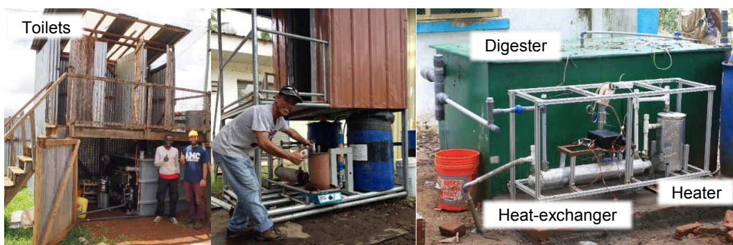
Figure 1.2 Installed ADPL systems in Kenya (left), Philippines (middle), and India (right).
